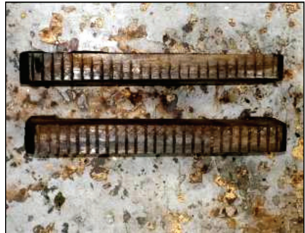
爪の摩耗状況、劣化度[a]
