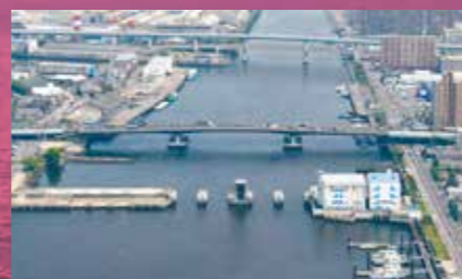
堀川口防潮水門 Tide gates at Horikawa River estuary
